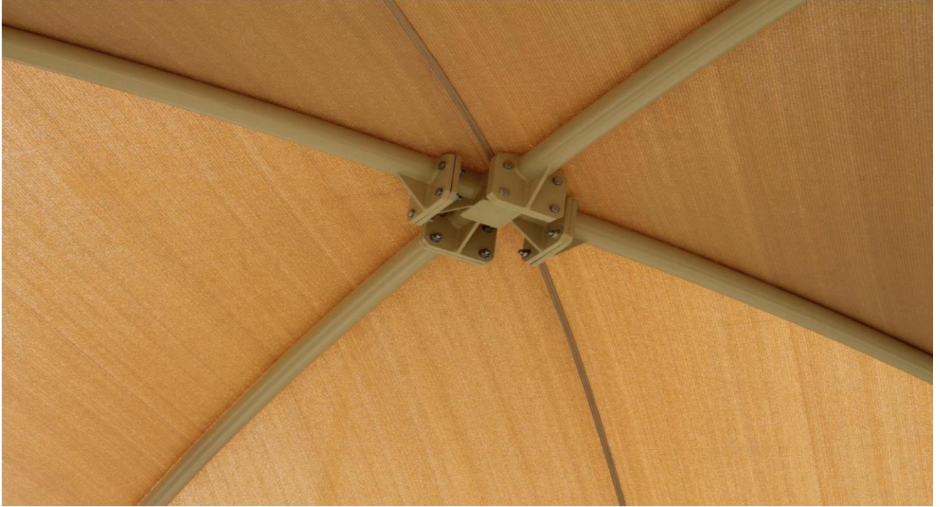
Car Parking Shade Top Section
