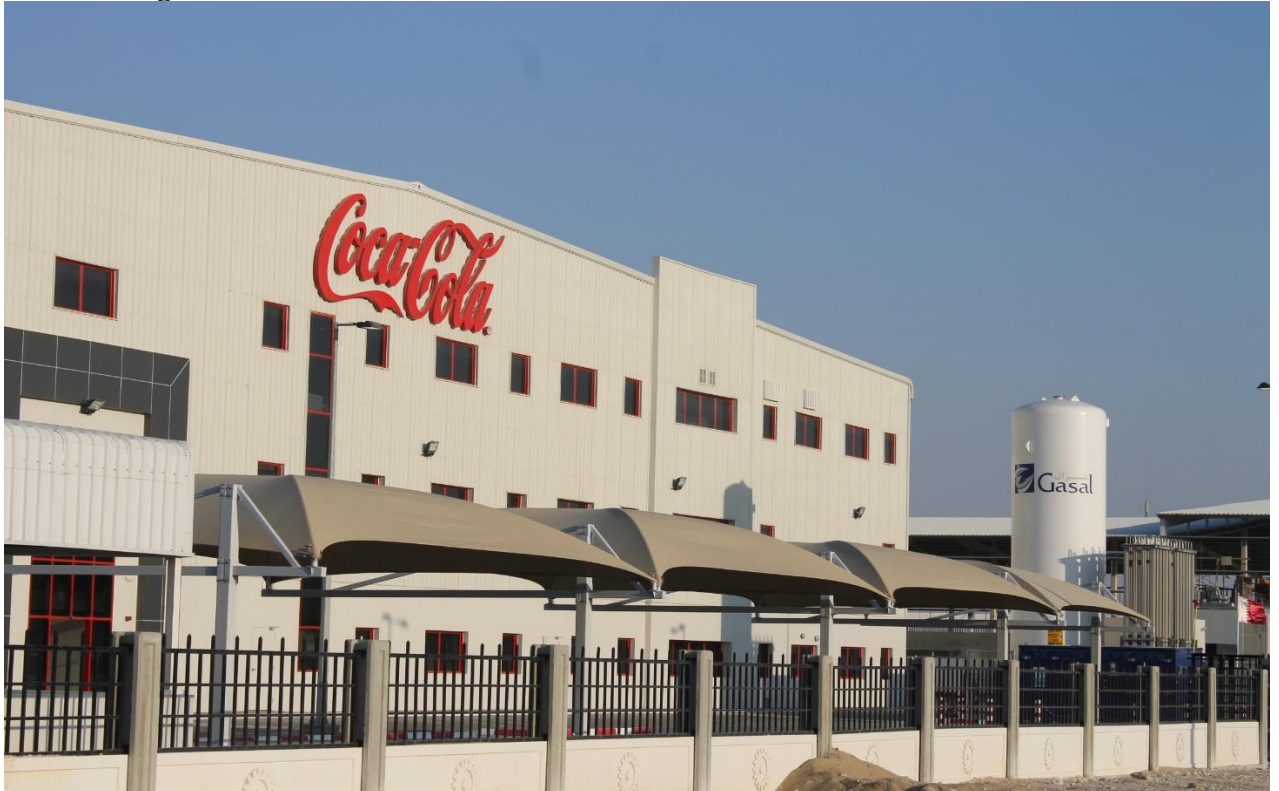
Car Parking Shade at Coca Cola Plant
