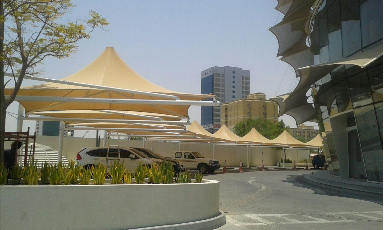
Car Parking Shade at Shiek Ghanem Business Center
