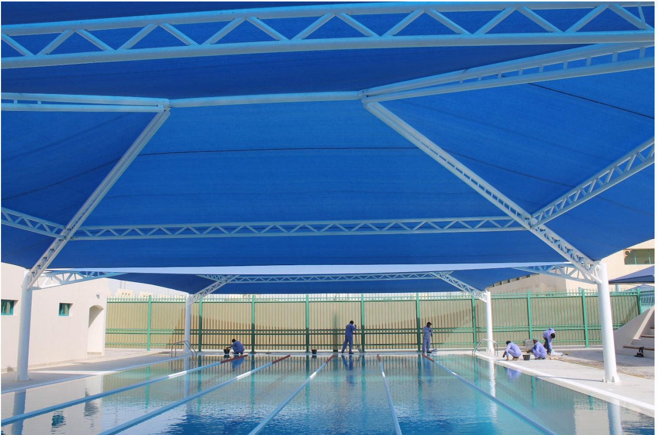
Swimming Pool Shade at Doha College
