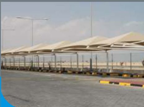
Car Parking Shade at GWC Rass Laffan
